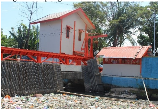
Gambar 2. Pos Pengoperasian Trashrack Kanal Jongaya.
